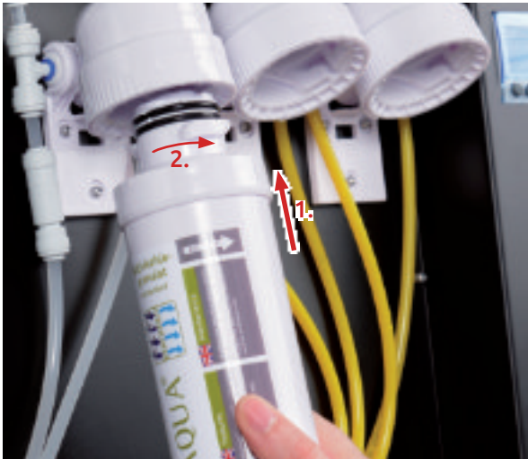
Lightly lubricate the O-rings of the new filter cartridges with petroleum jelly to facilitate installation and future replacement.
