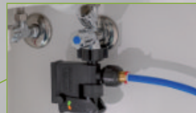
Blue 3/8" tube for water supply from the angle valve
