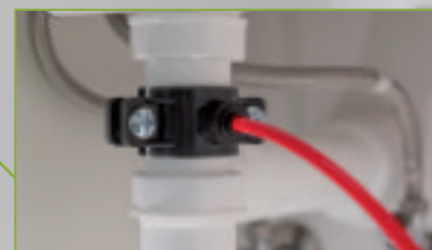
Red 1/4" tube for wastewater to the drain - maximum 2 meters
